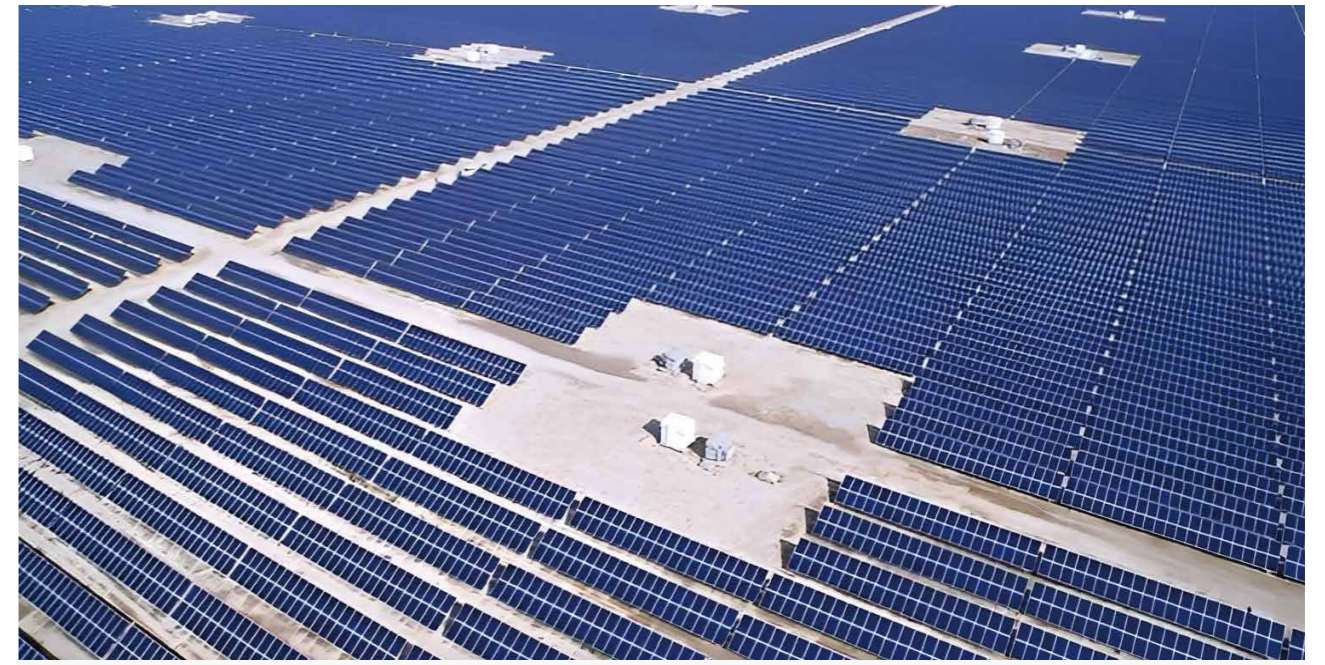
04 Utility Project in the Pakistan 900MW PV Plant
