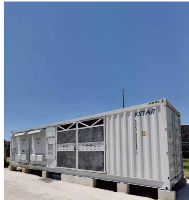
03 Utility Project in the Spain 10MW PV Plant
